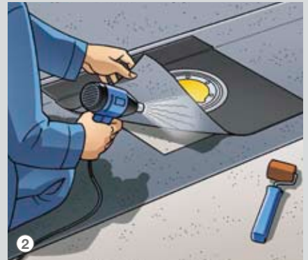
2 The EPDM side of the sealing collar is facing upwards. The collar is welded to the pre-laid sealing channel using hot air.
