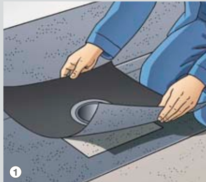
1 The dual-sided sealing collar (bitumen side up, EPDM side downwards) is placed over the drain and is tightly secured using the flange ring.
